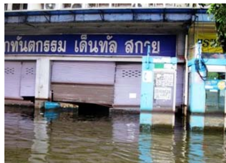
Standing water and damaged storefronts near Bangkok, where recent flooding has caused over 600 casualties. Photo Elizabeth Tromans/CRS
